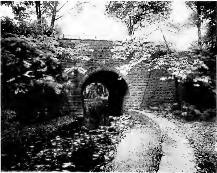
COUNTY BRIDGE AT RIDGEWOOD AVENUE
